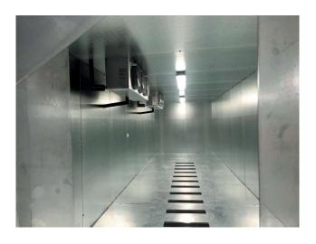
Handy Store Fixtures walk-in cooler and freezers set a new standard in high quality refrigeration room applications. Our Class 1 rated coolers and freezers feature tongue and groove cam locking wood frame construction, CFC-free urethane foam insulation, UL and NSF listed and approved, carrier rails for interior fittings, self-closing standard swing doors and other elements designed to improve the function and appearance of your refrigerated display units.
